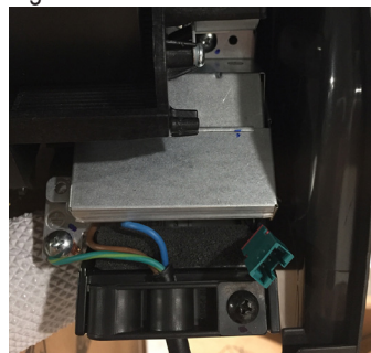
Figure 93: Terminal Cover Down.
