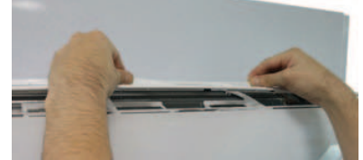
Figure 110: Disassembling the Air Filter (Appearances Will Vary Depending on Indoor Unit Model).
