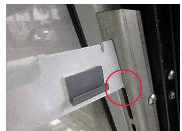
Bottom notch installed (no gap)
