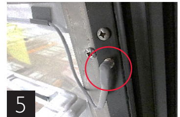
Light cord installed
