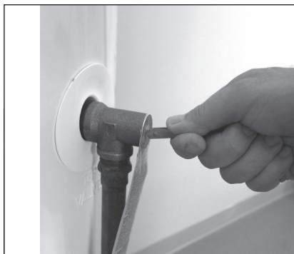
Figure 49 - T&P Relief Valve.
