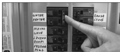
Figure 35 - Circuit Breaker.
