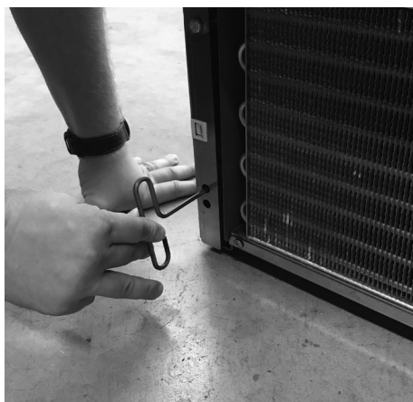
Adjusting rear leveling legs.
