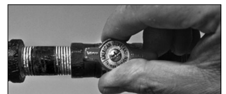
Figure 50 - Gas valve in "on" position.
