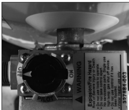
Figure 38 - Turn gas control knob OFF.
