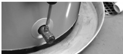
Figure 40 - Draining the water heater.
