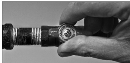
Figure 32 - Gas valve in "on" position
