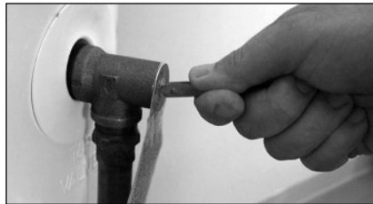
Figure 43 - T&P Relief Valve.
