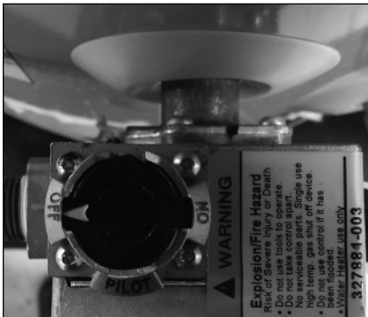
Figure 45 - Gas control/valve.
