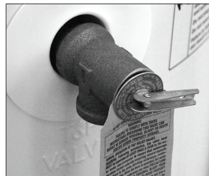
Figure 18: Temperature and Pressure Relief Valve
