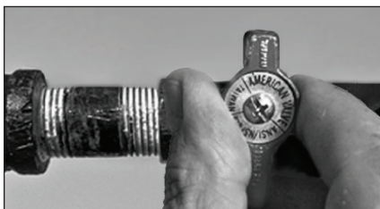
Figure 43: Gas valve in “off” position.
