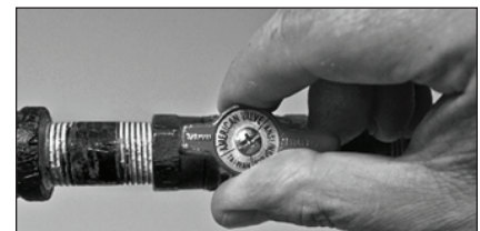
Figure 47: Gas valve in “on” position.
