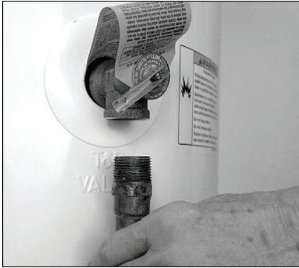
Figure 13: Removing the T&P Relief Valve discharge pipe.
