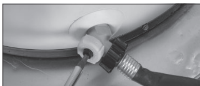
Figure 37: Draining the water heater.
