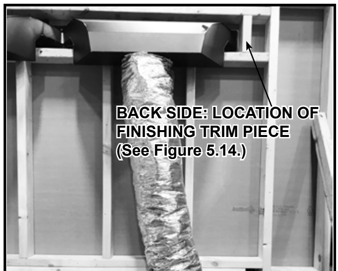
Figure 5.29 Flex Vent Installed with No Kinks
