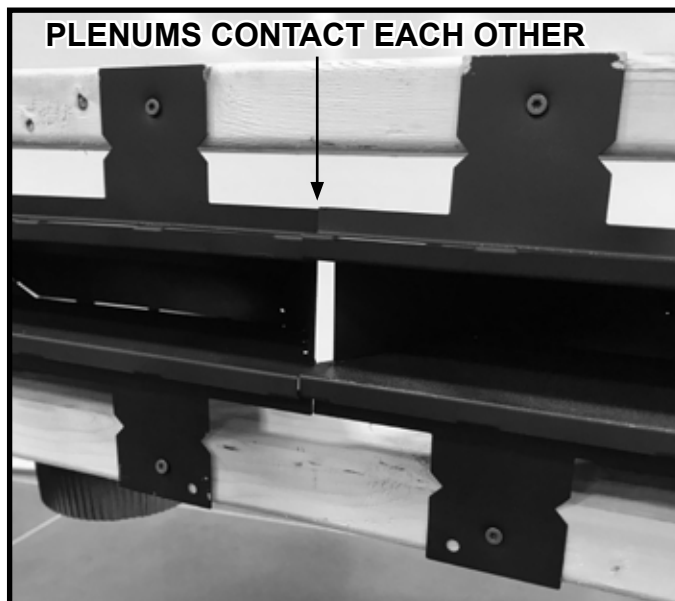
Figure 5.21 Plenums Contact Each Other
