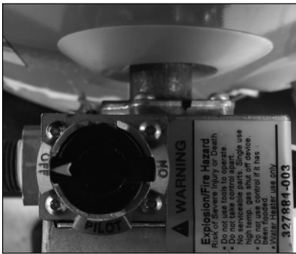
Figure 38 - Turn gas control knob OFF.
