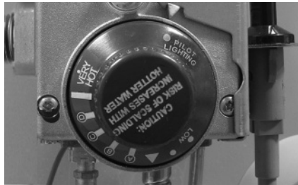
Figure 33 - Gas control/valve in Pilot Lighting position.
