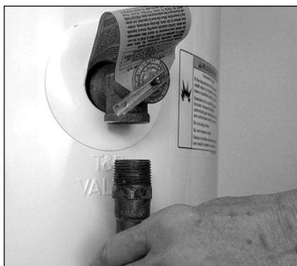
Figure 21 - Removing the T&P Relief Valve discharge pipe.
