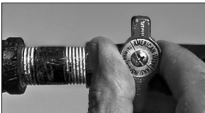
Figure 46 - Gas valve in "off" position.
