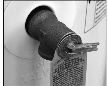
Figure 25 - Temperature and Pressure Relief Valve
