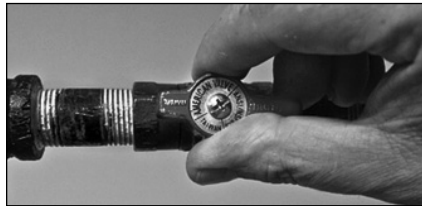
Figure 32 - Gas valve in "on" position
