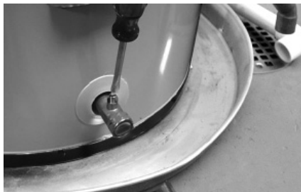
Figure 20 - Draining the old water heater.
