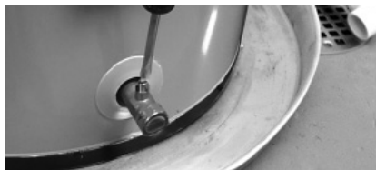
Figure 40 - Draining the water heater.
