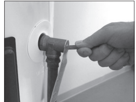
Figure 38 - T&P Relief Valve
