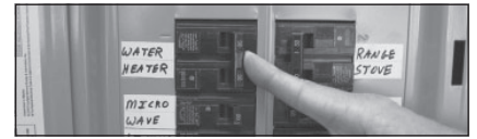
Figure 31 - Circuit Breaker
