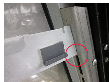
Bottom notch installed (no gap)
