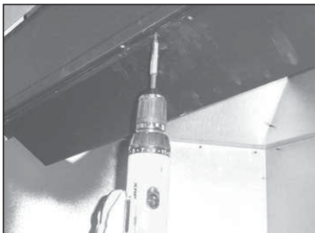
Figure 8.1 Remove Smoke Shield
