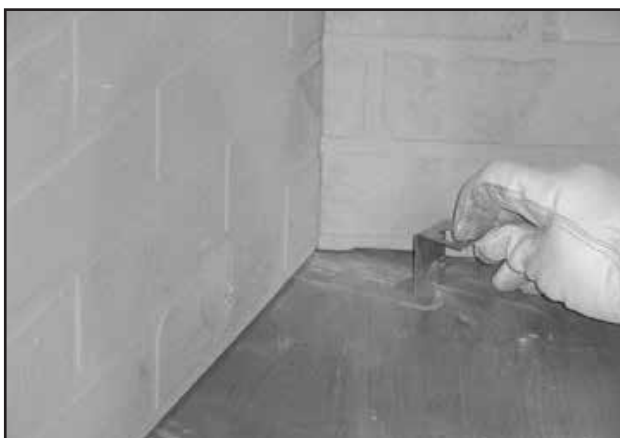
Figure 8.7 Slide Grate Retaining Bracket into Notch
